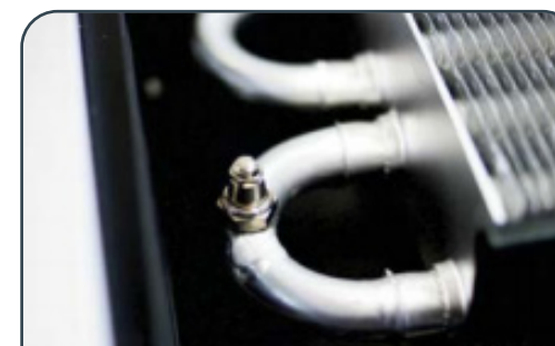
Air valve on heat exchanger
